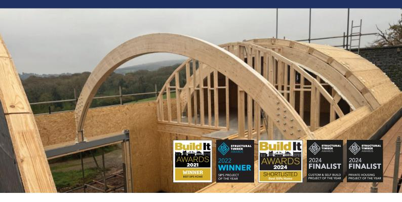
The structure is comprised of a hybrid SIP and steel frame construction and is asymmetric to adjoin the existing property. The walls are 142mm SIP panels and the roof is sectional 172mm SIP panels over large, curved Glulam beams.
