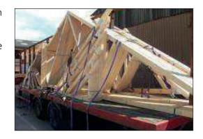
4. The manufacturer will supply truss packs secured to the trailer with 8mm blue rope. You should familiarise yourself with which rope attaches which pack to the centre bars.
