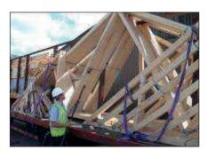
The crane will then lift the truss pack from the bed of the trailer. **NEVER** stand in the danger area where the trusses could potentially fall. Do not allow any others to enter the danger area.
