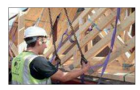
6. Once the order of unloading is agreed between the slinger and driver, the slinger will attach the purple lifting slings to the crane hooks.
