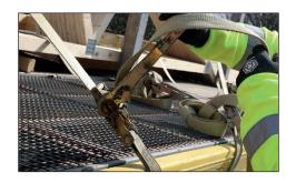
7. Ensuring the 8mm blue rope is holding the outer pack the driver will cut the company branded banding to allow separation of the individual trusses.
